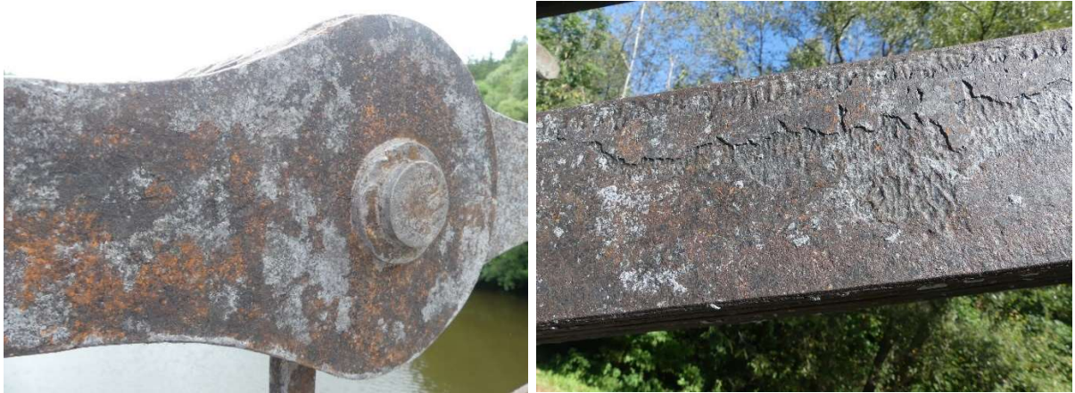
Figure 7 – Appearance of cleaned chain surface
