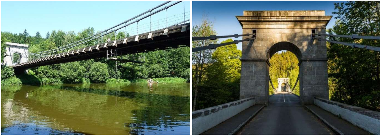
Figure 2 – Bridge construction cross Luznice near Stadlec
