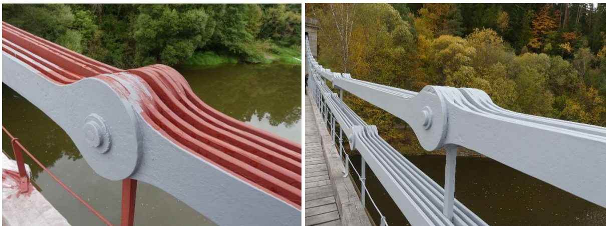
Figure 8 – Appearance of newly painted surface
